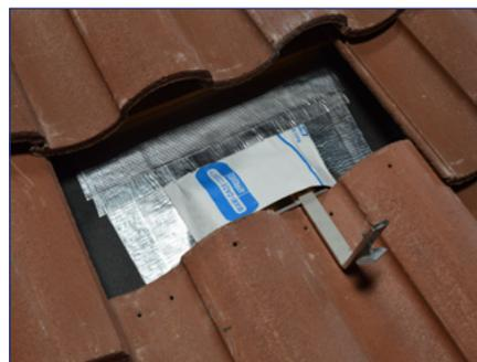
6) If deck-level flashing is required, integrate roof felt or a flexible flashing with the existing underlayment and over the Tile Hook.
