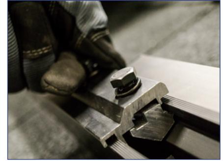
3) Lift up on splice insert to engage the upper lip of rail channel and tighten bolts by hand to secure insert in rails.
