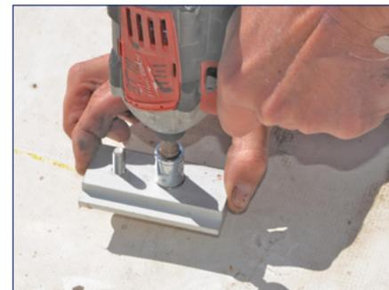
3) Attach the base with a 5/16" lag screw, drive lag screw for minimum 2.5" embedment into the roof framing member.
