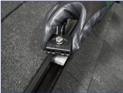
1) Snap Clamp into top or side rail channel.
