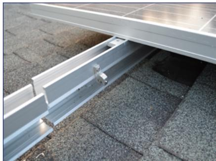
1) Drill and deburr a 1/4" hole in the back side of the rail for the IlSCO lug to attach to, place the bolt through the hole, and attach the lug assembly on **one rail per module row**.
