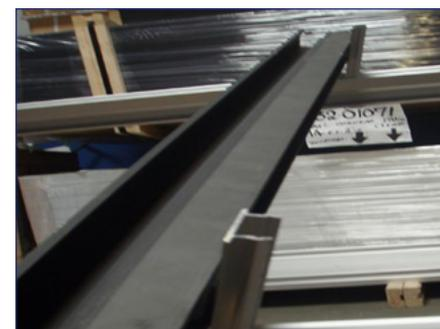
3) Adjust the rail covers to the correct positions, spaced at the same distance as that between the lower rail and top rail of tilted array.
