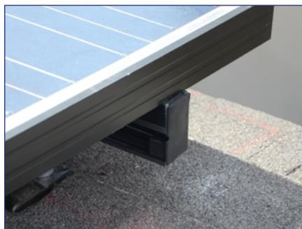
4) Insert SnapNrack Rail End Cap into the cut end of the rail to create a flush finish to the array.
