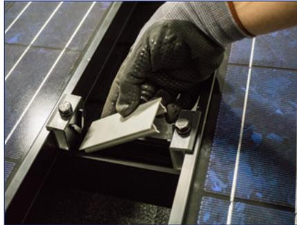
4) Snap Rail Cover into place, enclosing all conductors inside of rail channel.
