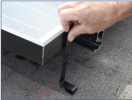
1) Measure required height of Array Edge Screen to determine which notch the clip will need to be broken off at.
