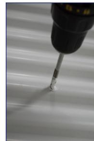
3) Attach the hanger bolt using the threaded bit adapter, drive hanger bolt for minimum 2.5" embedment of lag shank into the roof framing member.
