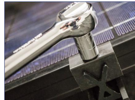
3) Tighten hardware, torque silver hardware to 10-16 ft-lbs and black hardware to 8-10 ft-lbs.
