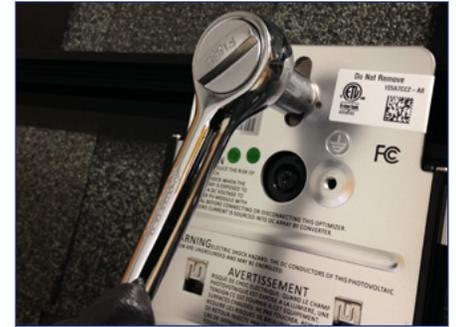
3) Tighten hardware, torque silver hardware to 10 ft-lbs.
