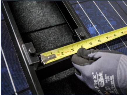
1) Measure the length of the SnapNrack 48" Rail Cover that is needed.
