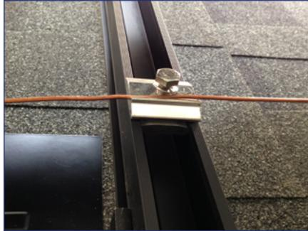
2) Place grounding conductor into the rail channel underneath split ring washer.
