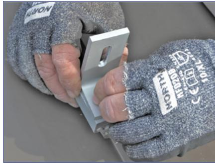
2) Attach the seam clamp to the standing metal seam by opening the seam clamp cam and placing the clamp over the top of the standing metal seam.
