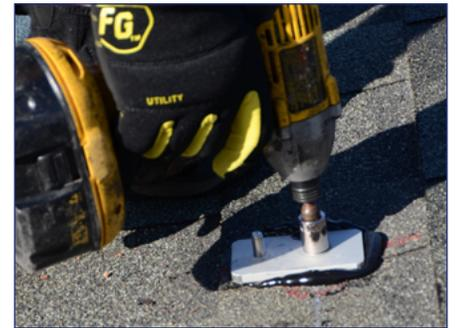
3) Attach the L Foot Base with a 5/16" lag screw, drive lag screw for minimum 2.5" embedment into the roof framing member.
