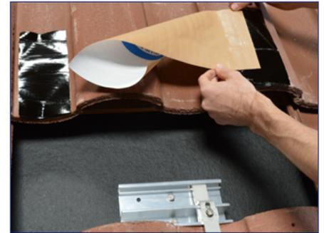
3) Apply the strips along the side edges of the synthetic underlayment flashing with 2" laps at the top and side edges.
