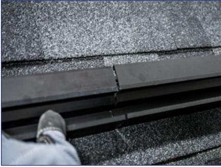
1) Align sections of rail so that ends butt up to each other.
