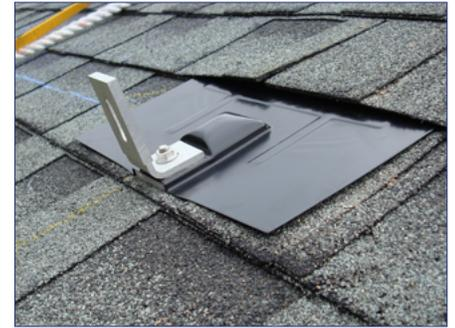
6) If necessary, adjust the vertical face of the L Foot with the "live hinge" feature and adjust angle of L Foot so that the vertical face is perpendicular to the roof surface.
