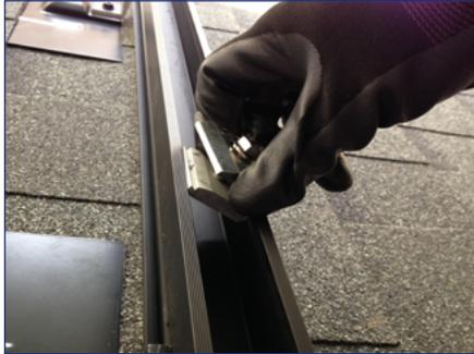
1) Snap the SnapNrack Ground Lug into the rail channel on **one rail per module row**.
