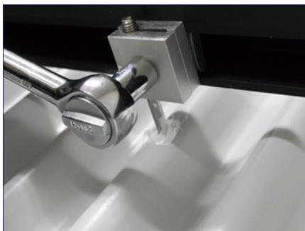
5) Attach the hanger bolt clamp by setting it around the threaded portion of the hanger bolt to the desired height and tighten to 10-16 ft-lbs.
