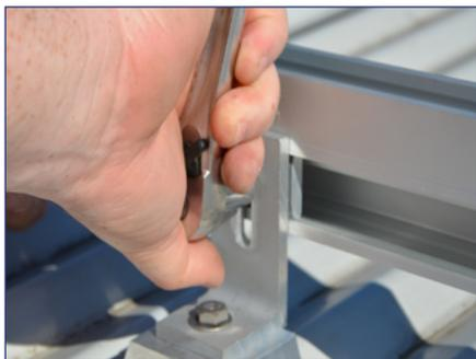
4) Install SnapNrack standard rail directly onto channel nut and tighten L Foot assembly silver hardware to 10-16 ft-lb.
