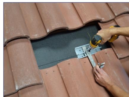
5) Once hook arm position is set, tighten the bolt in the channel nut and ensure the arm fully seats to the base.
