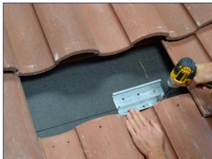
2) Apply roofing sealant and attach the base with (2) 5/16" lag screws, drive lag screws for minimum 2.5" embedment into the roof framing member.
