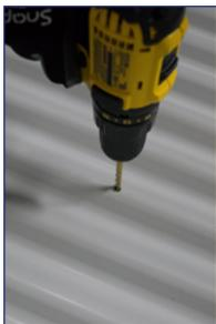
1) Using roof attachment locations drawn during system layout, drill a pilot hole through the roofing material into the roof framing member.
