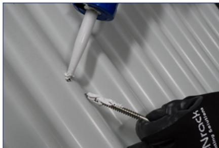
2) Apply roofing sealant directly onto the pilot hole and the hanger bolt to ensure a water tight seal.
