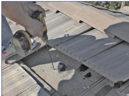
1) Using roof attachment locations drawn during system layout, remove roof tile where the roof attachment will be installed and drill a pilot hole through the roofing material into the roof framing member.
