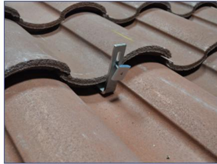
7) Replace the roof tiles and install SnapNrack Standard Rail directly to the available channel nut on the hook arm.
