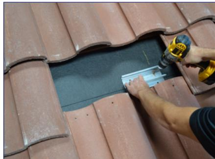
1) Using roof attachment locations drawn during system layout, remove roof tile where the roof attachment will be installed and drill two pilot holes through the roofing material into the roof framing member.
