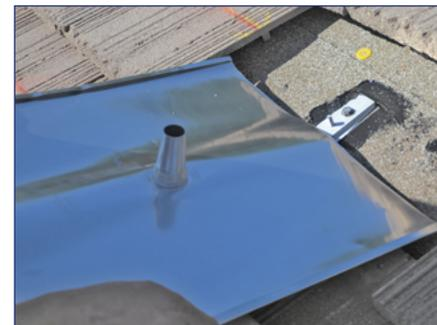
3) Set the flashing by sliding the flashing underneath the row of tiles directly above the installed base, with the hole in the flashing directly above the base stud.
