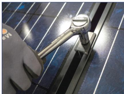
4) Tighten hardware, torque silver hardware to 10-16 ft-lbs and black hardware to 8-10 ft-lbs.
