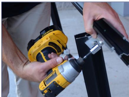
6) For tilts greater than 15 degrees, cut length of rail to use as rear tilt leg and attach to rear standoff using L Feet hardware.
