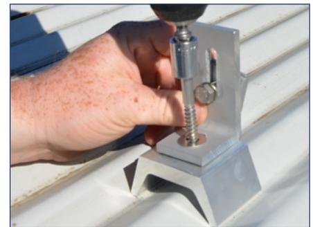
3) Attach the Straddle Block and L Foot with 5/16" lag screw, drive lag screw for minimum 2.5" embedment into the roof framing member.
