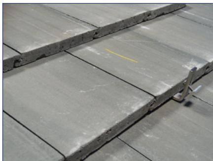
4) Replace the roof tiles and install SnapNrack Standard Rail directly to the available channel nut on the hook arm.
