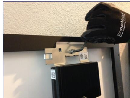
2) Install the optimizer mounting plate onto the module frame and tighten the socket cap screw to 10 ft-lbs.
