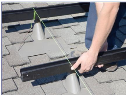
5) Level the remaining rails to the string line by working out from the middle rail, add leveling spacers if needed.
