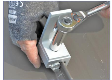
3) Torque black seam clamp bolt to 200 in-lbs (16.7 ft-lbs).
