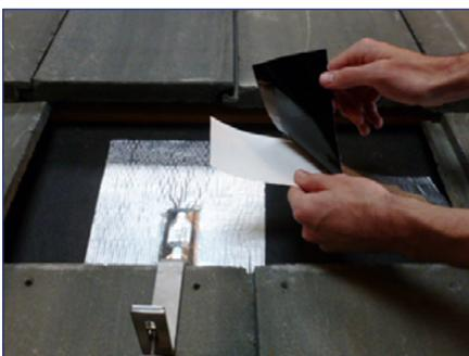
5) Peel off the backing from a 4" by 13" strip of flexible flashing.
