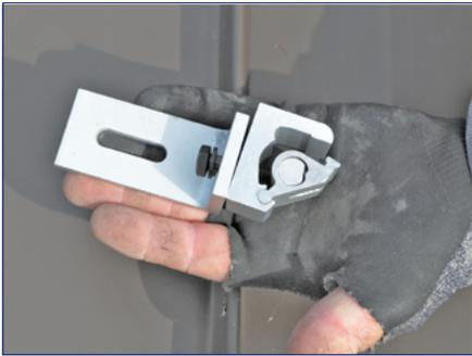
1) Loosen seam clamp hardware and use roof attachment locations to lay out seam clamps on roof.
