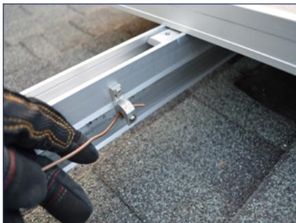
2) Place grounding conductor into slot.
