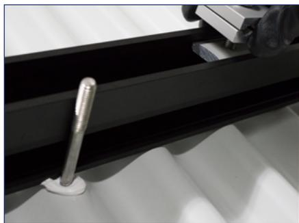
4) Attach the channel nut of the hanger bolt assembly into side channel of rail.
