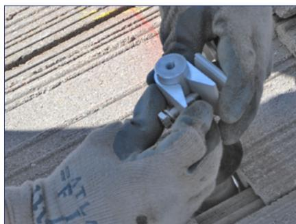
5) Cut the tile to fit around the flashing, replace the tile, then attach the standoff clamp by first sliding the rubber rain collar over the standoff shaft then the standoff clamp with bolt, washer and channel nut.
