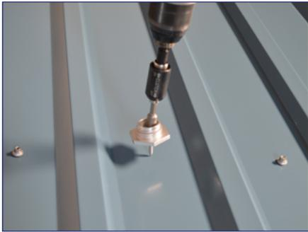
1) Using roof attachment locations drawn during system layout, drill a pilot hole through the roofing material into the roof framing member.
