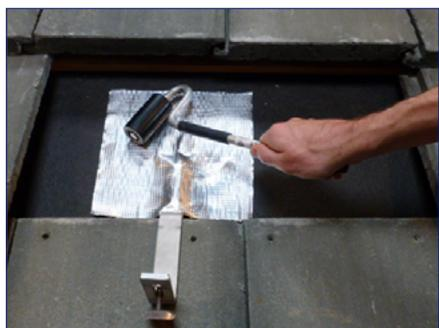
4) Press and smooth out any creases or air bubbles with a roller to maximize contact of the flashing adhesive to 100% of the surface and Tile Hook.
