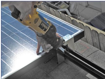
2) Use the reciprocating saw or band saw to cut off the end of the rail.
