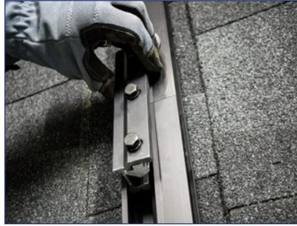
2) Set rail splice assembly in to the side channel of rail, making sure the base is seated all the way into the channel and that the splice is centered.
