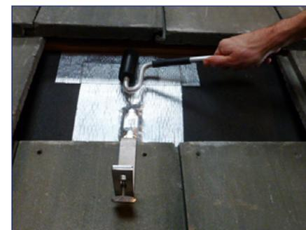
6) Apply the strip with 2" laps at the top and side edges of the square flashing. Roll out any creases or air bubbles between the strip, the flashing and the underlayment surface.
