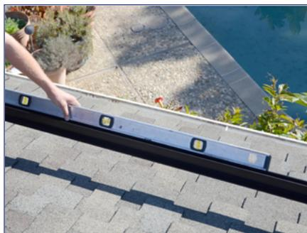
2) Level the bottom rail of the array to the roof and tighten attachment points, silver hardware to 10-16 ft-lbs and black hardware to 8-10 ft-lbs.
