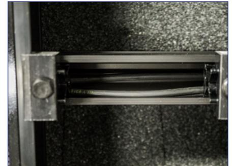
3) Place all electrical conductors in the bottom of the rail channel.
