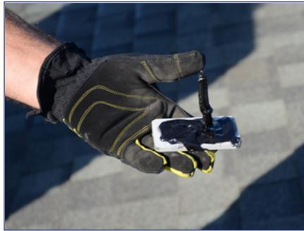
2) Apply roofing sealant to the bottom of the base and directly onto the lag screw to ensure a water tight seal.
