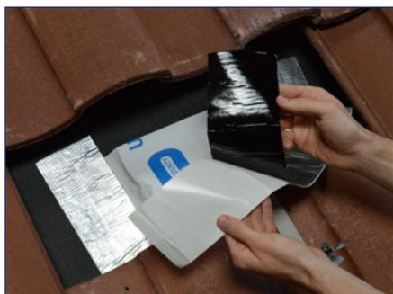
6) Peel off the backing from a 4"x19" strip of flexible flashing.
