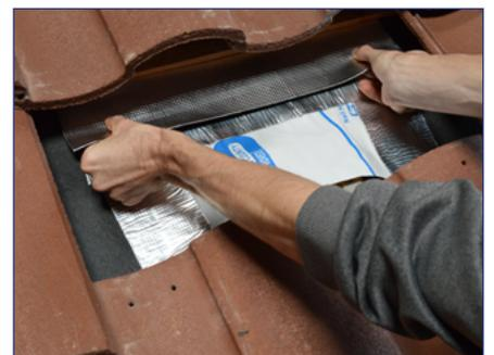
8) Peel off the backing and apply the second 4"x19" strip of flexible flashing along the top edge of the first strip with a 2" lap at the top edge, then roll out any creases between the strip and the deck-level surface.
