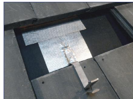
3) If deck-level flashing is required, integrate roof felt or a flexible flashing with the existing underlayment and over the Tile Hook.
