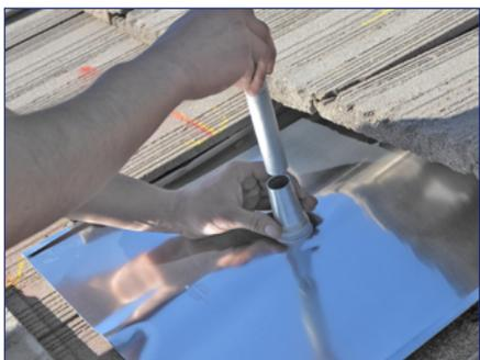
4) Attach the standoff shaft by sliding it through the hole in the flashing and tighten it onto the base stud with channel locks.
