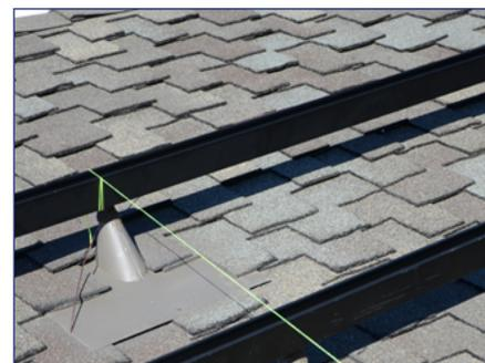
3) Run a string line or spare rail from the bottom rail to the top rail and set desired pitch of the array by adjusting the top rail, add leveling spacers if needed.
