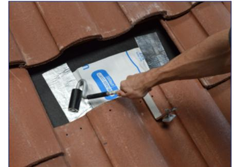
5) Press and smooth out any creases or air bubbles with a roller to maximize contact of the adhesive to 100% of the flashing and deck-level surface.
