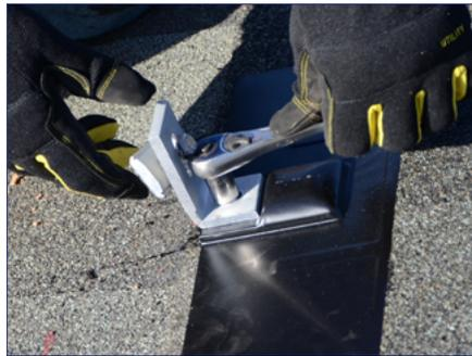
5) Place the L Foot on the base stud over the flashing and tighten the flange nut over the L Foot, torque to 10 - 16 ft-lbs.
