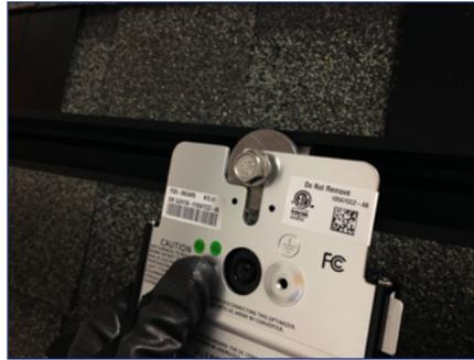
2) Install the microinverter mounting plate onto the bolt of the MLPE Rail Attachment Kit, ensuring that the large fender washer is between the rail and mounting plate.
