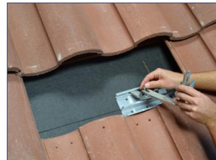
3) Insert the top end of the arm into the groove at the top of the base and slide the arm to position it over the valley of the tile below, then lower the arm down.
