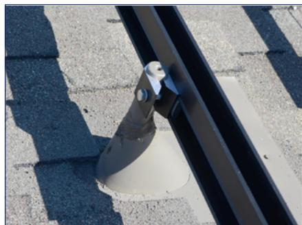
1) Set rails into the attachments by snapping channel nuts into the side channel of the rail. Connect multiple lengths of rail end to end using the SnapNrack rail splice.
