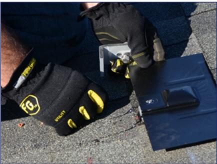
4) Pry up shingles with a breaker bar and install flashing underneath shingle course above installed base, position flashing so base stud extends through hole in bottom edge of flashing.
