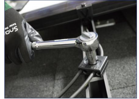
3) Tighten Wire Clamp with 1/2" socket, ensure cables and conductors are aligned in the clamp slots.
