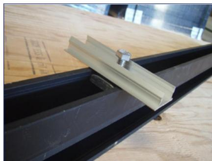
2) Assemble bolts and channel nuts in rail covers through the pre-drilled holes with channel nut on flat side of rail cover, then slide or snap channel nuts into top channel of rail.
