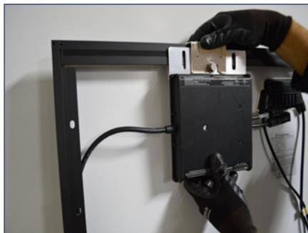
2) Slide the microinverter unit onto the bracket clamp, then move it slightly to the left.
