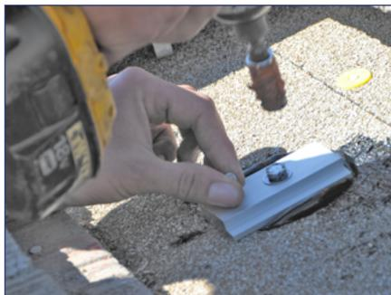
2) Apply roofing sealant and attach the base with a 5/16" lag screw, drive lag screw for minimum 2.5" embedment into the roof framing member.
