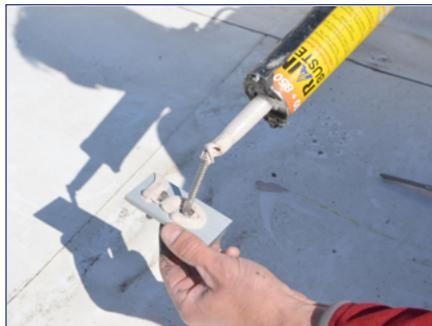
2) Apply roofing sealant directly onto the pilot hole and the lag to ensure a water tight seal.
