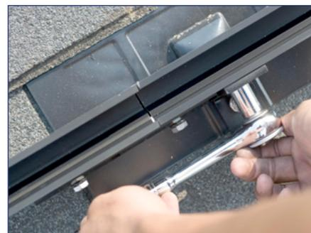
6) Tighten all racking hardware, silver hardware to 10-16 ft-lbs and black hardware to 8-10 ft-lbs.
