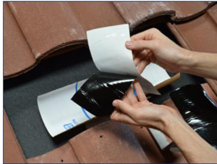
2) Peel off the backings from two 4"x8" strips of flexible flashing.
