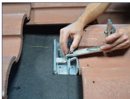
4) Work the channel nut into the lower groove of the base as you lower the arm, without removing the channel nut.
