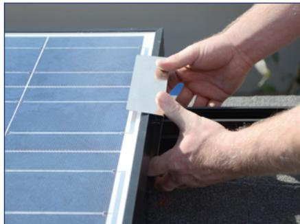
1) Slide the Rail Cutting Tool over the end of the rail and place it so that the upper lip is safely covering the edge of the module.
