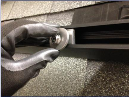
1) Snap the SnapNrack MLPE Rail Attachment Kit channel nut into the desired location on the rail where the microinverter will be installed.
