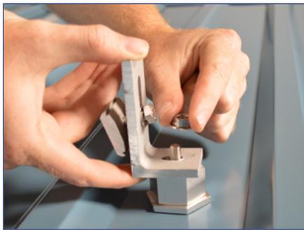
4) Attach L Foot to stud in Metal Roof Base cap.
