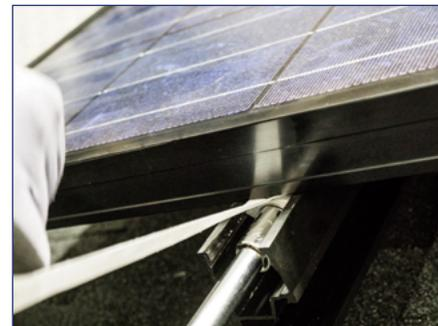
3) Use the pull tab to hold the UEC taut towards the end of the rail and tighten hardware to 10 - 16 ft-lbs.
