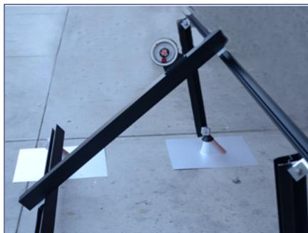
7) Set array tilt and tighten hardware to 10-16 ft-lbs.
