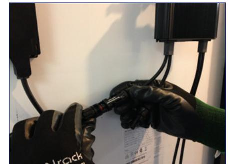
3) Connect the module leads to the input connectors on the optimizer.
