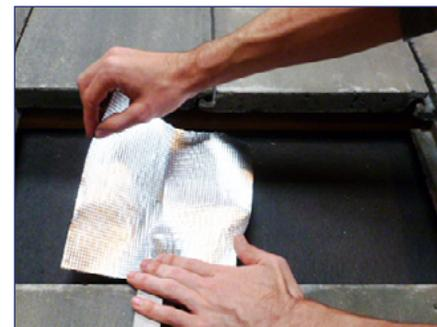
3) Apply flexible flashing centered laterally over tile hook and abutted to the tile hook arm.
