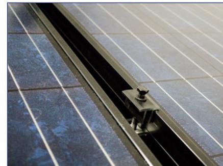
3) Place the next module flush to the other side of the mid clamp.
