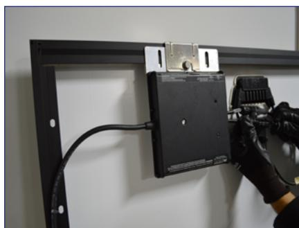
4) Connect the module leads to the microinverter DC connectors.
