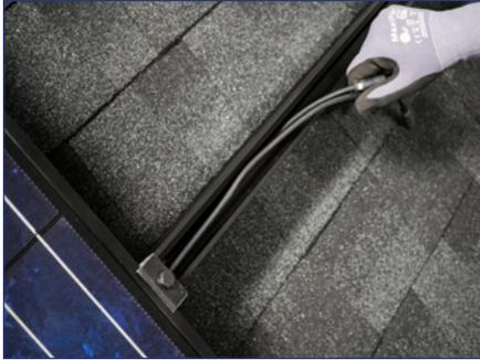
1) Place all electrical conductors in the bottom of the rail channel.
