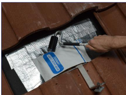
7) Apply the strip along the top edge of the flashing with 2" laps at the top and side edges, then roll out any creases or air bubbles between the strip, the flashing, and the deck-level surface.
