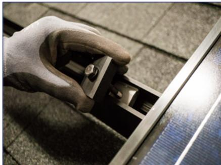
1) Snap the channel nut into the top channel of the rail.
