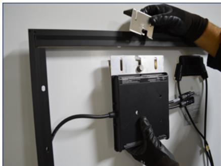
1) Locate the Enphase Frame Mount bracket clamp at a location on the module frame that will not interfere with the SnapNrack rail.
