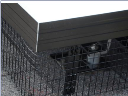
4) Slide the Array Edge Screen into the hooks on the Edge Screen Clips and repeat for all locations around the array.
