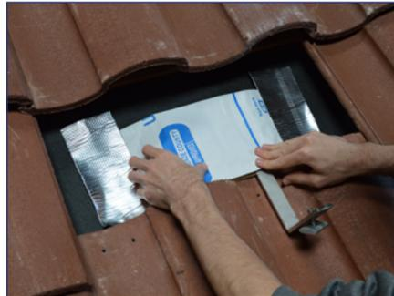
4) Apply the synthetic underlayment flashing centered over the tile hook and abutted to the lower row of tile.
