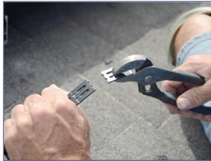
2) Use pliers to break the Array Edge Screen Clip at the appropriate length.
