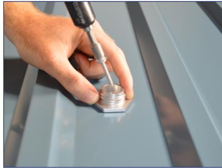
2) Attach the base with 5/16" lag screw (or 1/4" self-drilling screw), drive lag screw for minimum 2.5" embedment into the roof framing member.
