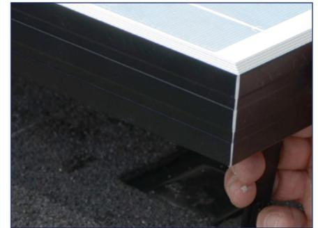
3) Clip the Array Edge Screen Clip to the lip on the underside of the modules around the area that the edge screen will be installed.
