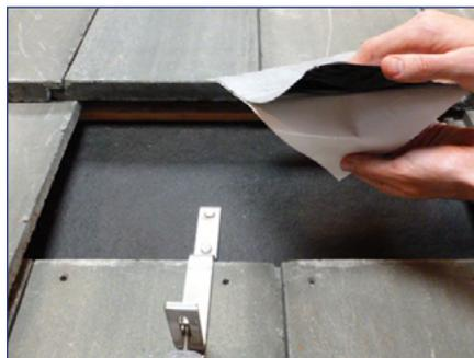
2) Peel off the backing from a 9" square of flexible flashing.
