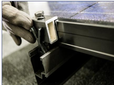
2) Slide the clamp flush to the module with the top lip of the end clamp over the top edge of the module frame.
